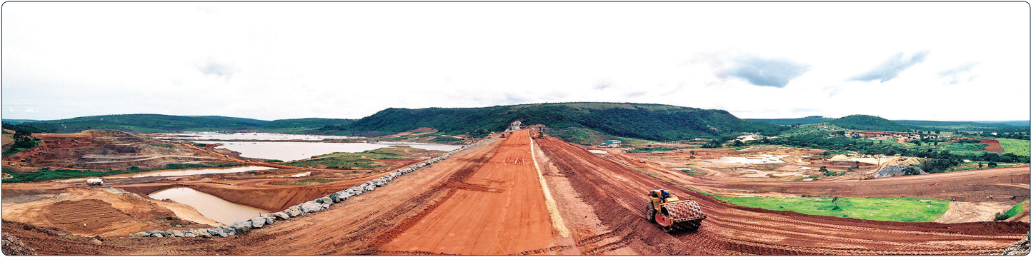
Panoramic view of an earthfill dam under construction.
