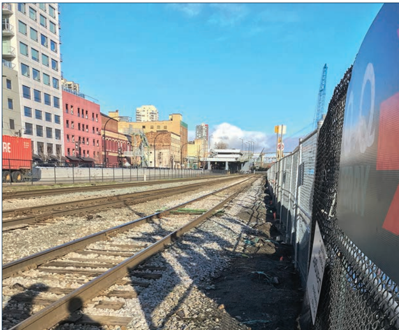
Three rail tracks run alongside the construction site.
