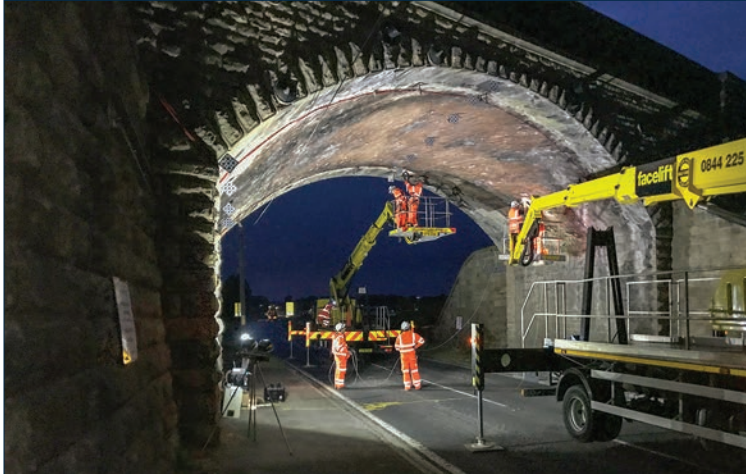
A boom lift was used during non-peak hours for installation of the instrumentation.
