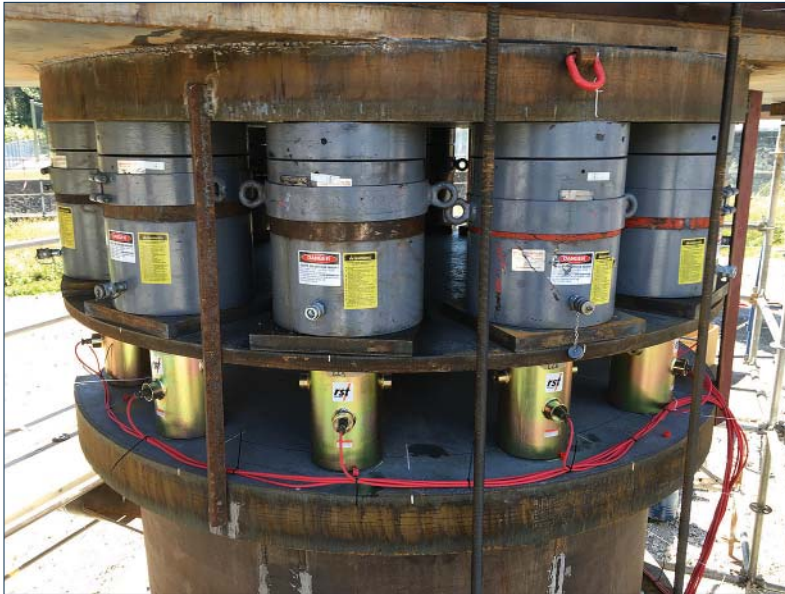
High Capacity Strain Gauge Load Cells and Hydraulic Jacks ready for the test.
