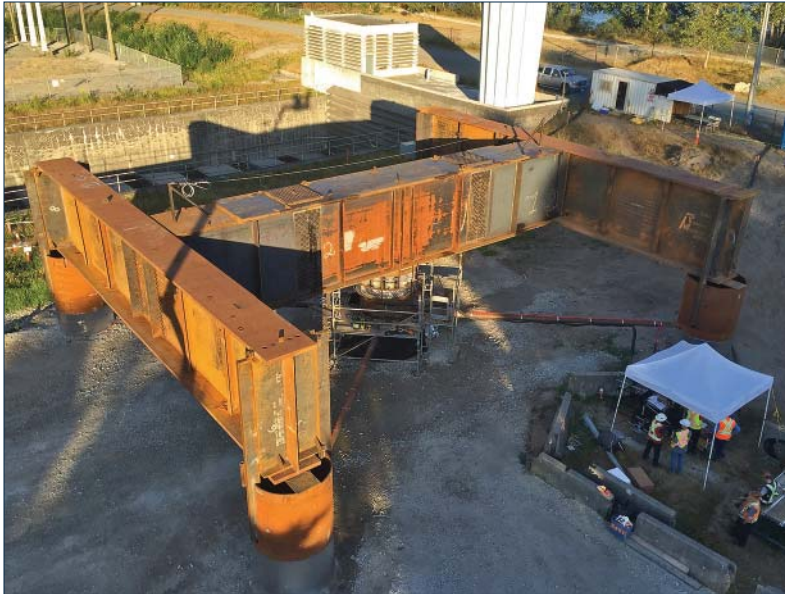
Pile test setup with Massey Tunnel entrance in background.
